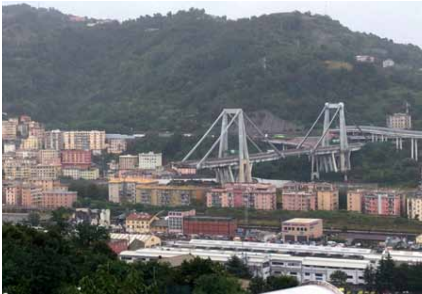
The Morandi Bridge in Genoa, Italy, in August 2018, after its collapse. There are no spans in the foreground.
