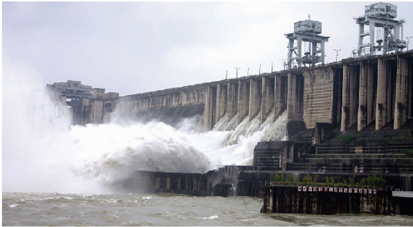
The Danjiangkou Dam on the Han River, the principal reservoir for the middle line of the South-to-North Water Diversion Project, was heightened to increase its impoundment volume, over a construction period from 2005 (shown here) to 2010. The dam was raised 14.6 m, from 162 m to 176.6 m.
