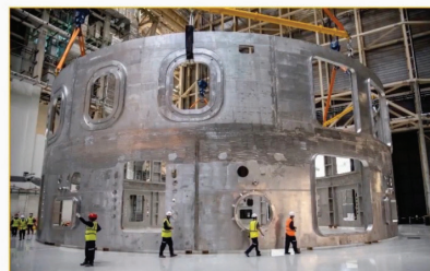
Cryostat Lower Cylinder lift 31 August 2020
