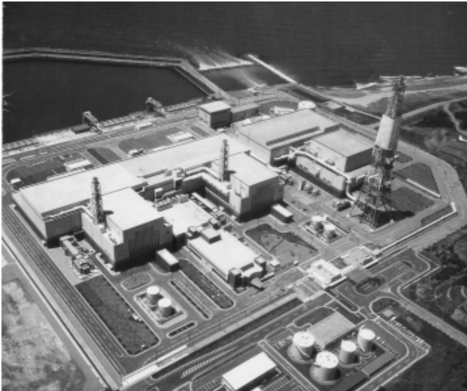
This General Electric ABWR design was built in Japan by Hitachi and Toshiba, for Tokyo Electric Power Co., putting two units of 1,356 megawatts each on line at the Kashiwazaki-Kariwa site in Japan in record time in 1997 and 1998.
