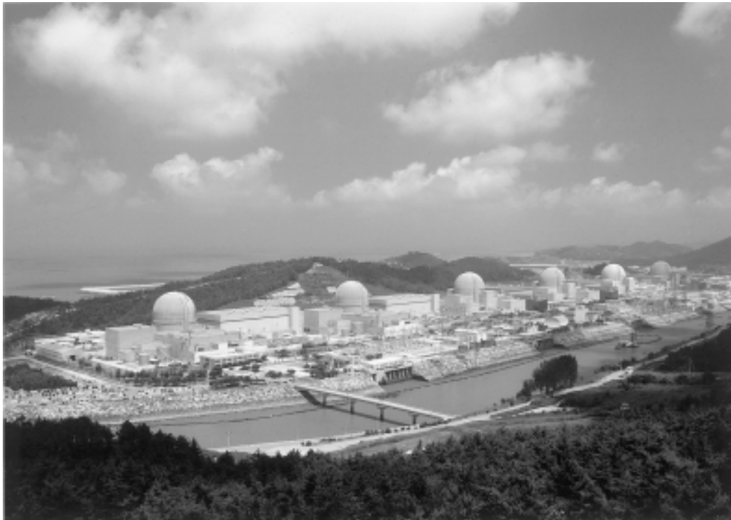
South Korea's Yongwang nuclear complex with six reactors.
