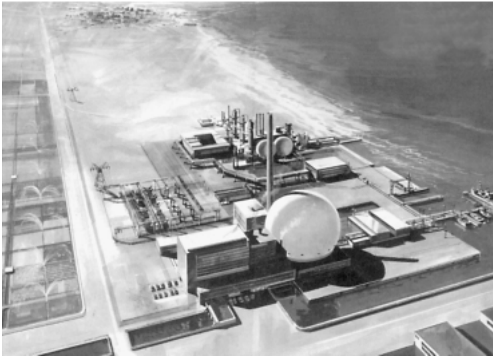
Nuclear energy will be used for many applications, such as desalination of seawater. This 1960s sketch is of a nuplex, an agro-industrial complex centered on a nuclear power plant. It is located on the seacoast, making possible the large-scale irrigation of farmland.
