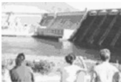
Here LYM members contemplate the magnificent construction of the Grand Coulee Dam.
