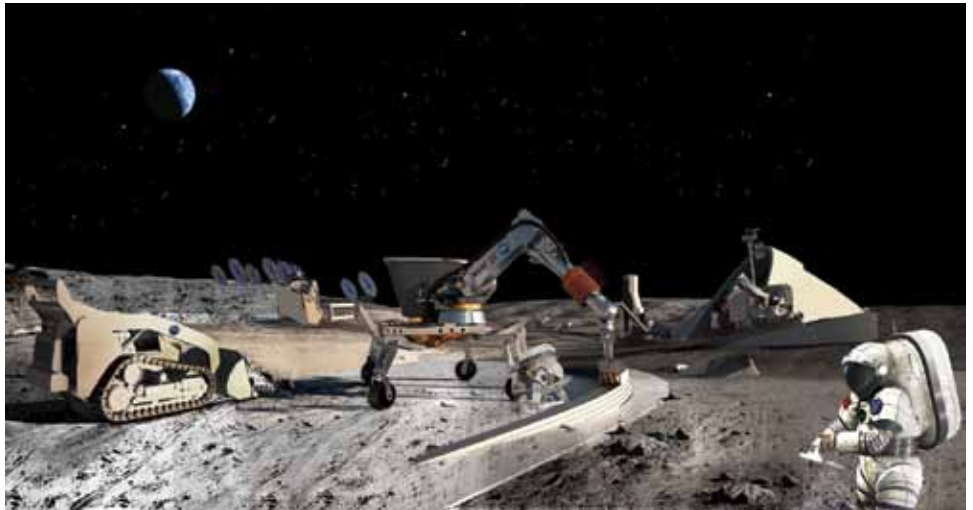
Artist’s concept for a lunar base built through in-situ resource utilization (ISRU) and a form of 3D printing known as contour-crafting.
