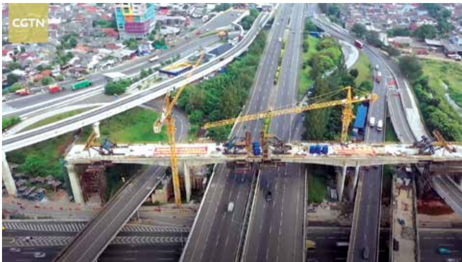
Box girders are emplaced in the construction of an overpass for Indonesia's 142 km Jakarta-Bandung High-Speed Railway. This Belt & Road project was 79% complete as of Nov. 2021.
