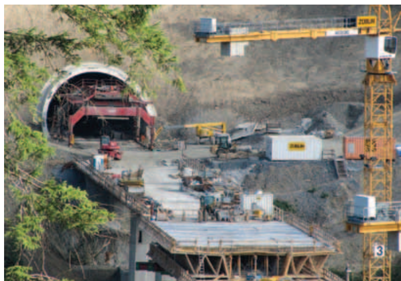
BRI has not been stopped by Pompeo. A tunnel under construction in Indonesia.
