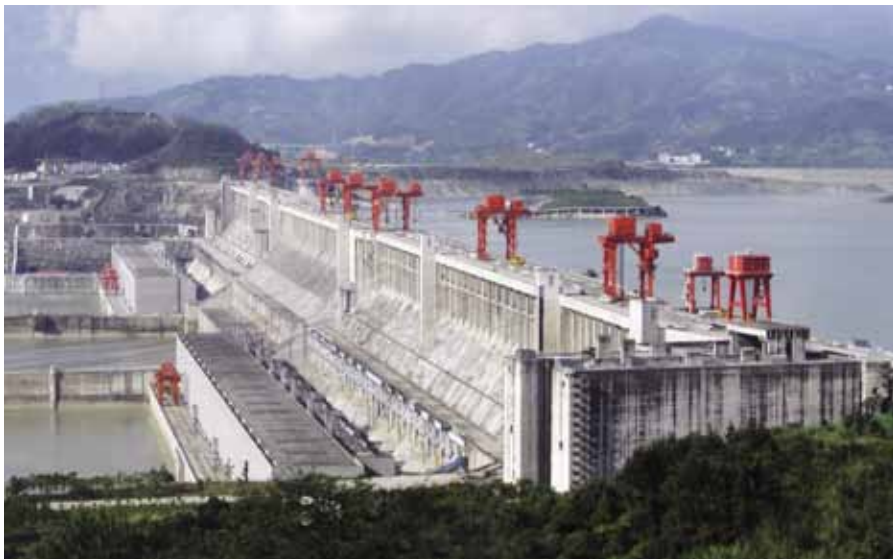
The Three Gorges Hydroelectric Dam on the Yangtze River, Hubei province, China.
