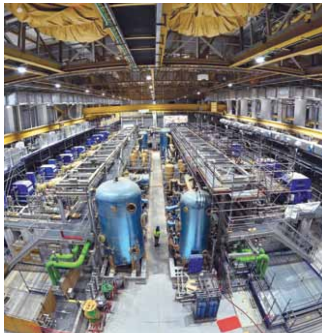
ITER The cryoplant provides cooling fluids to ITER, the world’s largest magnetic confinement plasma physics experiment, in France.
