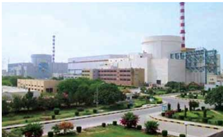
The Chinese-supplied unit 4 pressurized water reactor at Chashma is Pakistan's fifth nuclear power plant.
