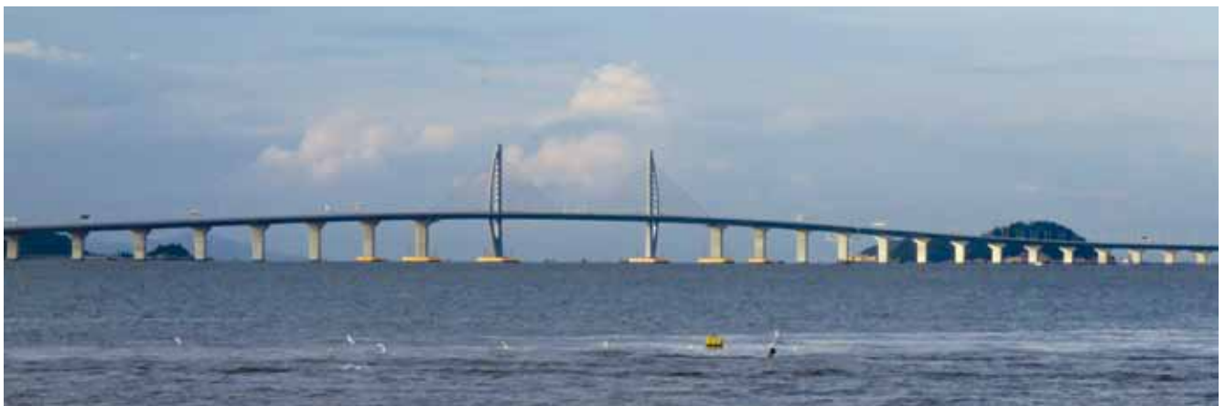
The West section of the Hong Kong-Zuhai-Macau Bridge in 2018.
