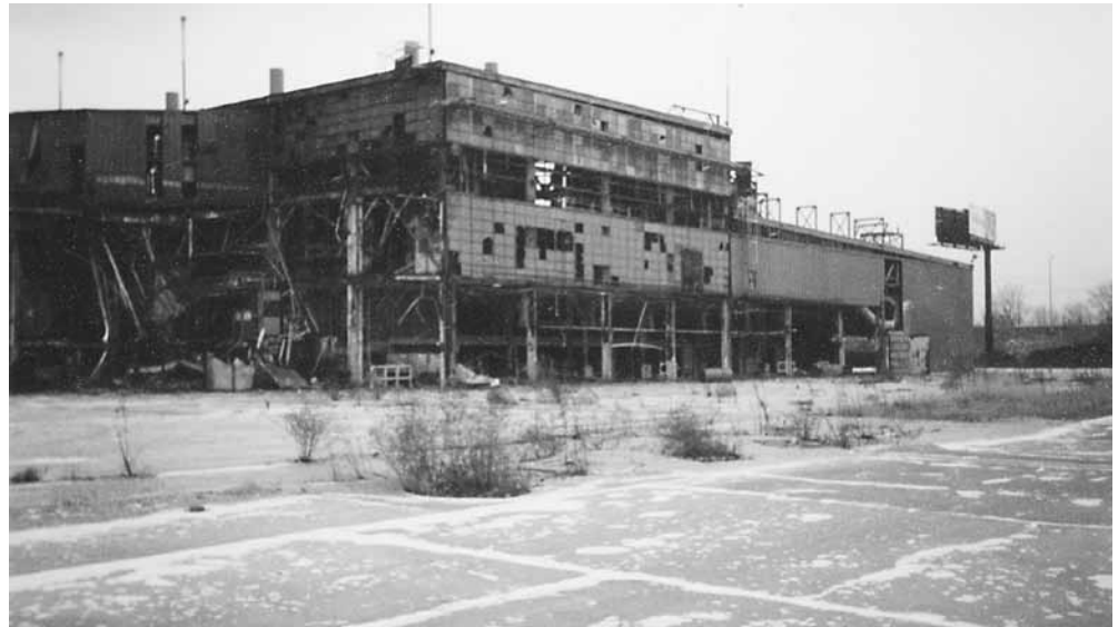
Abandoned GM plant, Danville, Illinois.
