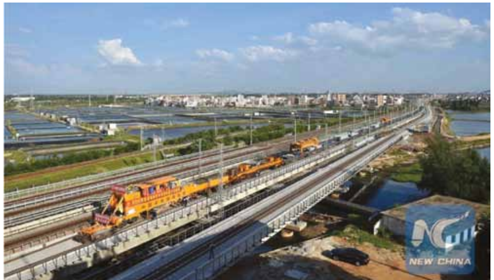
A track-laying vehicle lays the last section of steel rail on the western ring of the high-speed rail loop line, in south China’s Hainan Province, June 30, 2015.
