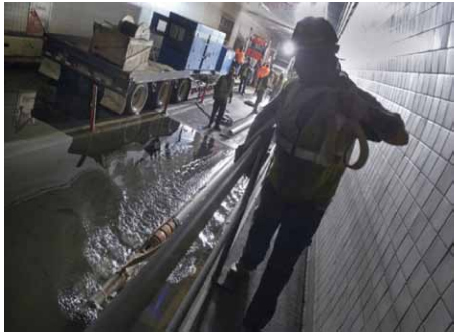
Flooded subways after Hurricane Sandy: MTA Bridges and Tunnels workers pumping 43 million gallons of water out of each of the tubes of the Brooklyn-Battery Tunnel.
