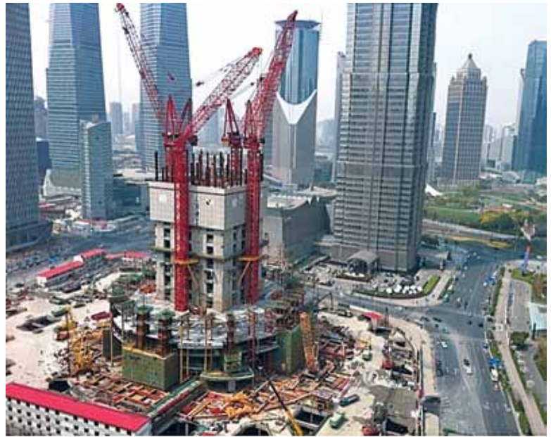
Shanghai Tower under construction, April 12, 2011.
