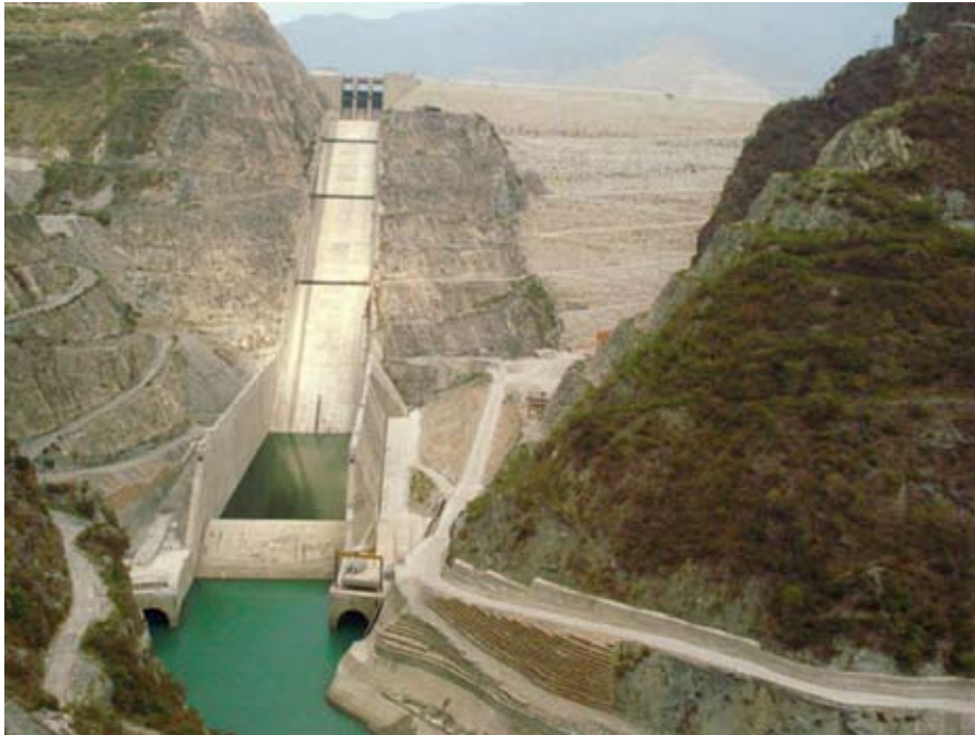
Tehri Dam/Arvind Iyer
