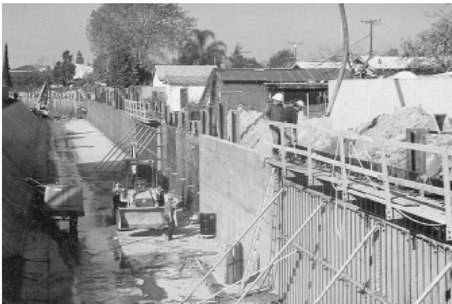
“The great and crucial portion of the new capital-formation in basic economic infrastructure, will be as international capital associated with long-term treaty agreements among sovereign nation-states.” Here, a U.S. Army Corps of Engineers project for construction of a retaining wall at Sargent Beach, Texas, on the Gulf of Mexico.
