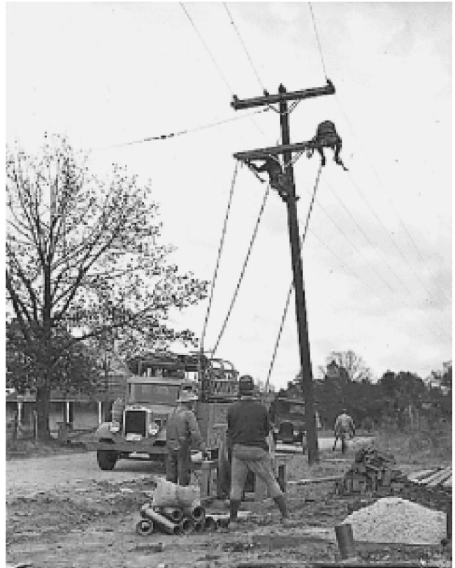
Franklin Roosevelt's Rural Electrification Act had incomparable effects on the productivity of U.S. agriculture. This shows electrical wire being strung in rural areas where the TVA was producing power.
