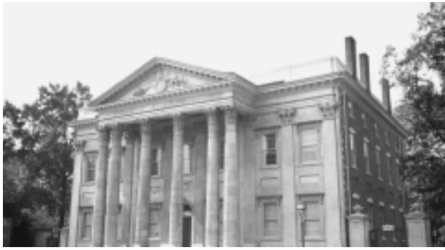
The First National Bank of the United States, which Hamilton fought to establish as a means of providing credit for industrial development, was located in Philadelphia, and still stands today.
