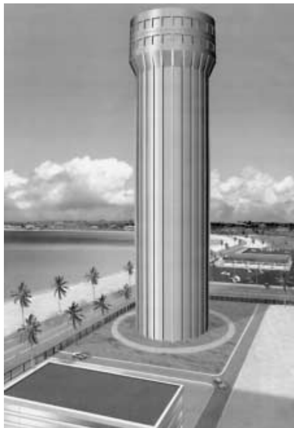
Artist's depiction of a modern seawater desalination tower. It is proposed for a location on the Pacific Coast of California. The structure houses a multi-effect distillation process (vertically stacked evaporators) for large-scale output (284,000 cubic meters daily).
