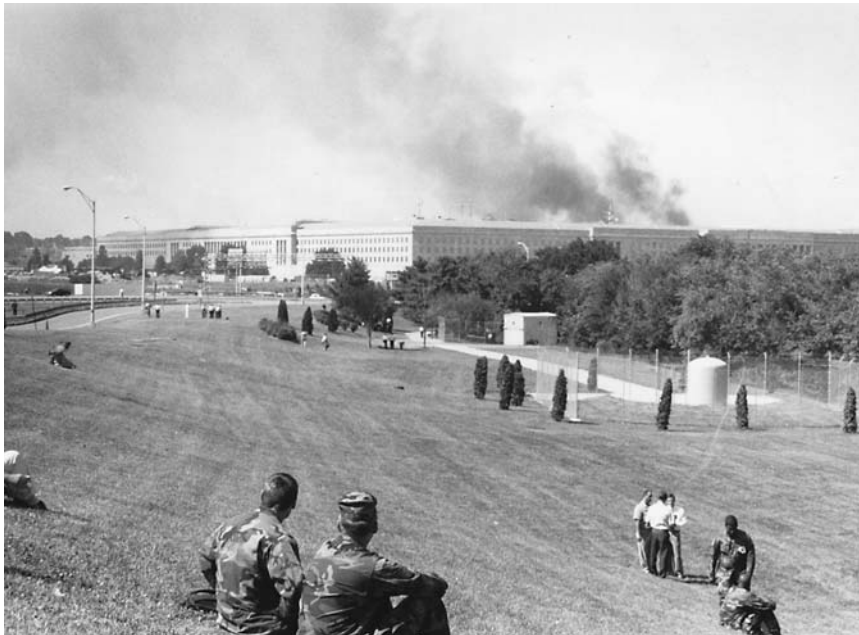
The Pentagon in flames, shortly after a hijacked airliner was crashed into the building on Sept. 11.
