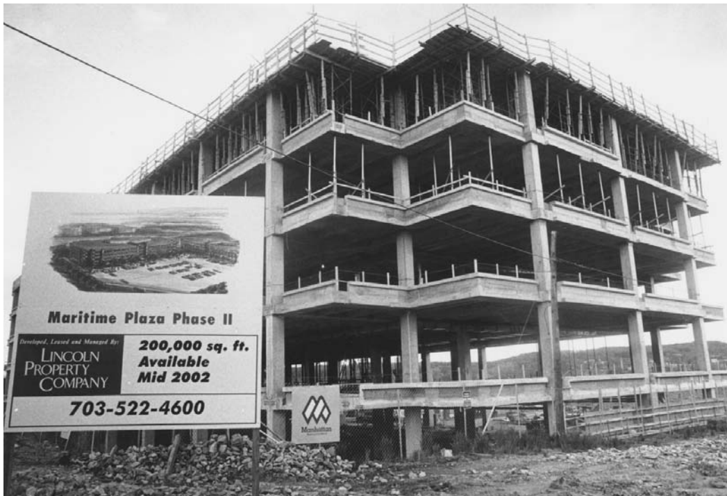
Office building construction in Southeast D.C., in the triangular area just east of the Navy Yard; according to the Washington Business Journal, it is hoped that this project, along with others, “could help build the momentum for a major transformation of this historically underdeveloped area.”
