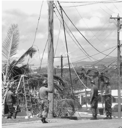
Repairing downed power lines.
