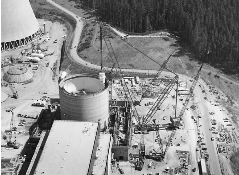
Part of the 5,000 megawatts of nuclear power capacity, partly built and then abandoned and never put on line, which could have been providing power to the West Coast states from Bonneville Power Authority and Washington Public Power.
