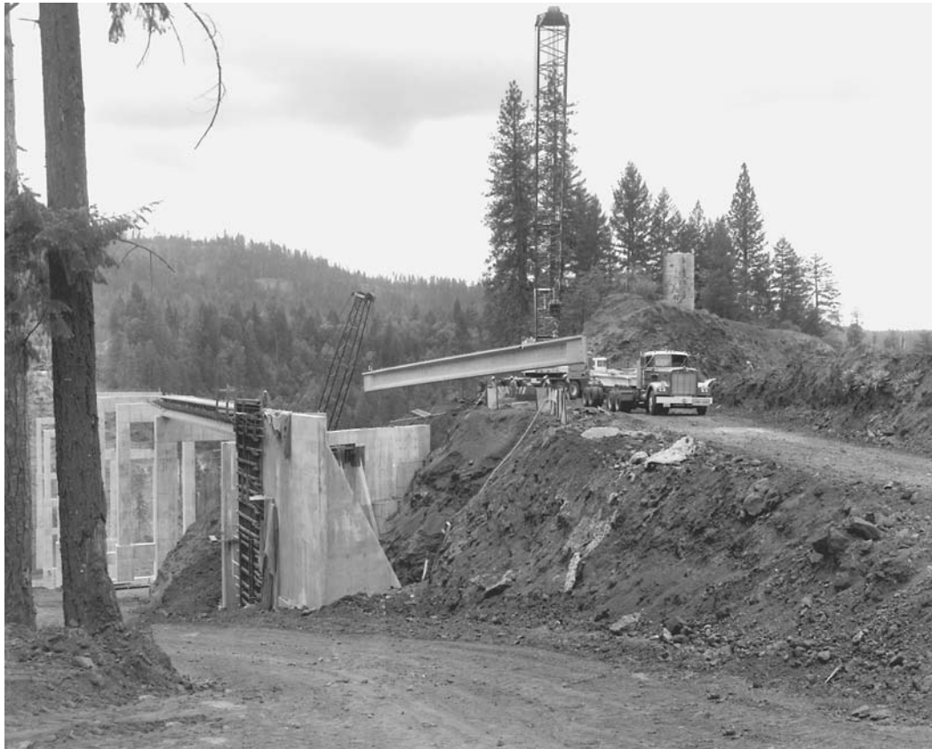
The U.S. Army Corps of Engineers works on a bridge project at Lost Creek Lake, Oregon. The Corps has a vital role to play, with cooperating non-military agencies, in conducting a large-scale development of the basic economic infrastructure of our nation, and in cooperation with other nations.
