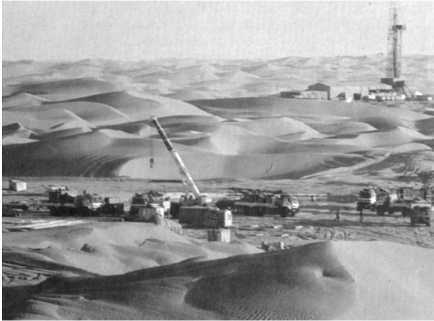
An oil well in the Taklimakan Desert in China. The area is an important reserve base of China's oil resources.
