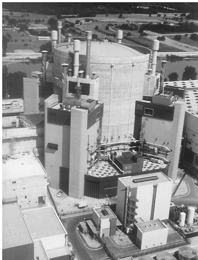
The core of the Superphénix reactor, while under construction. This vital project has been halted, thanks to an agreement between the Socialist Party and the Greens.
