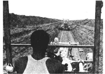
Building a canal in Rahad, Sudan.
