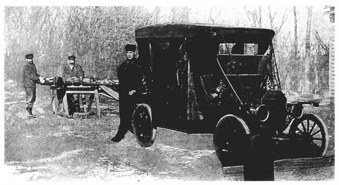
The Ford Model-T could be rapidly changed into a traveling saw-mill. Henry Ford conceived the Model-T to be used as a universal farm machine.
