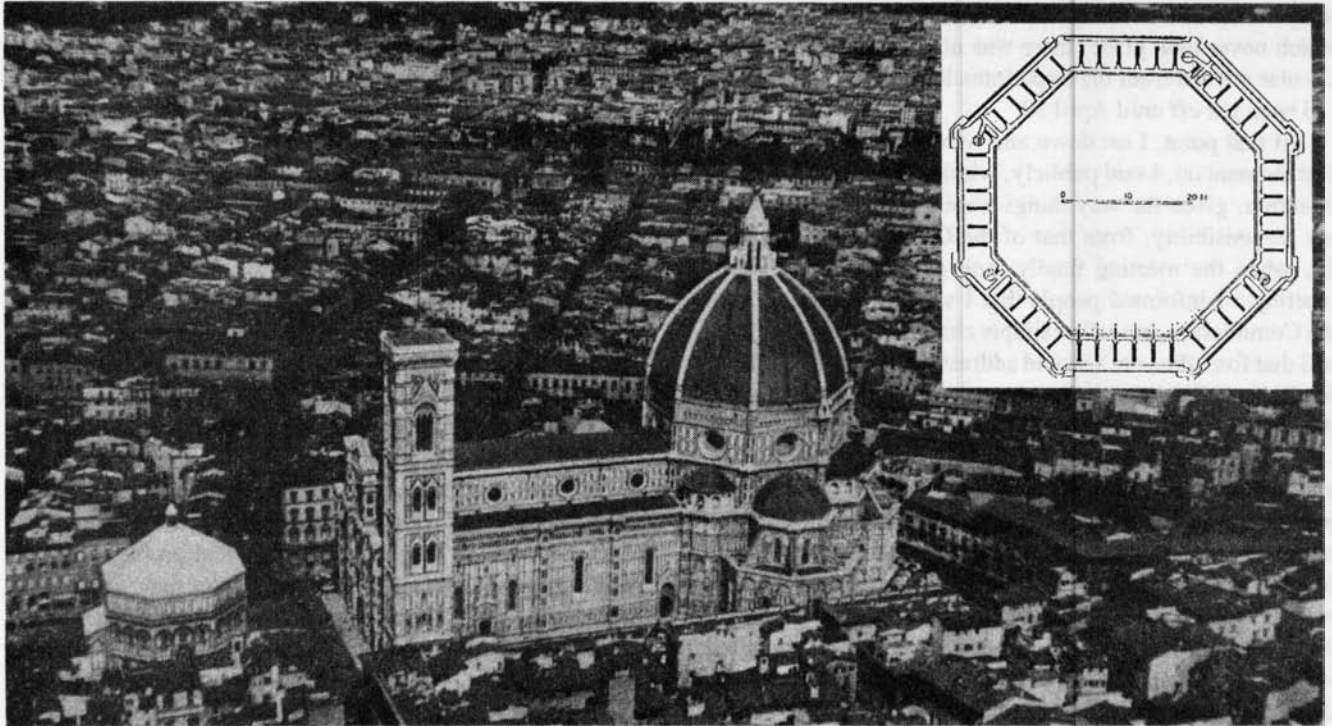
Brunelleschi's dome in its Florentine setting. Inset: Plan of the 48 staging holes left open by the architect at the base of the cupola, to support scaffolding for maintenance work, and allow the cupola to "breathe."
