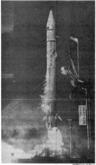
General Dynamics built the first American ICBM, the Atlas. In 1961, the Atlas carried the first American into orbit. The Atlas launch shown here carried the Centaur upper-stage rocket developed by Krafft Ehricke.
