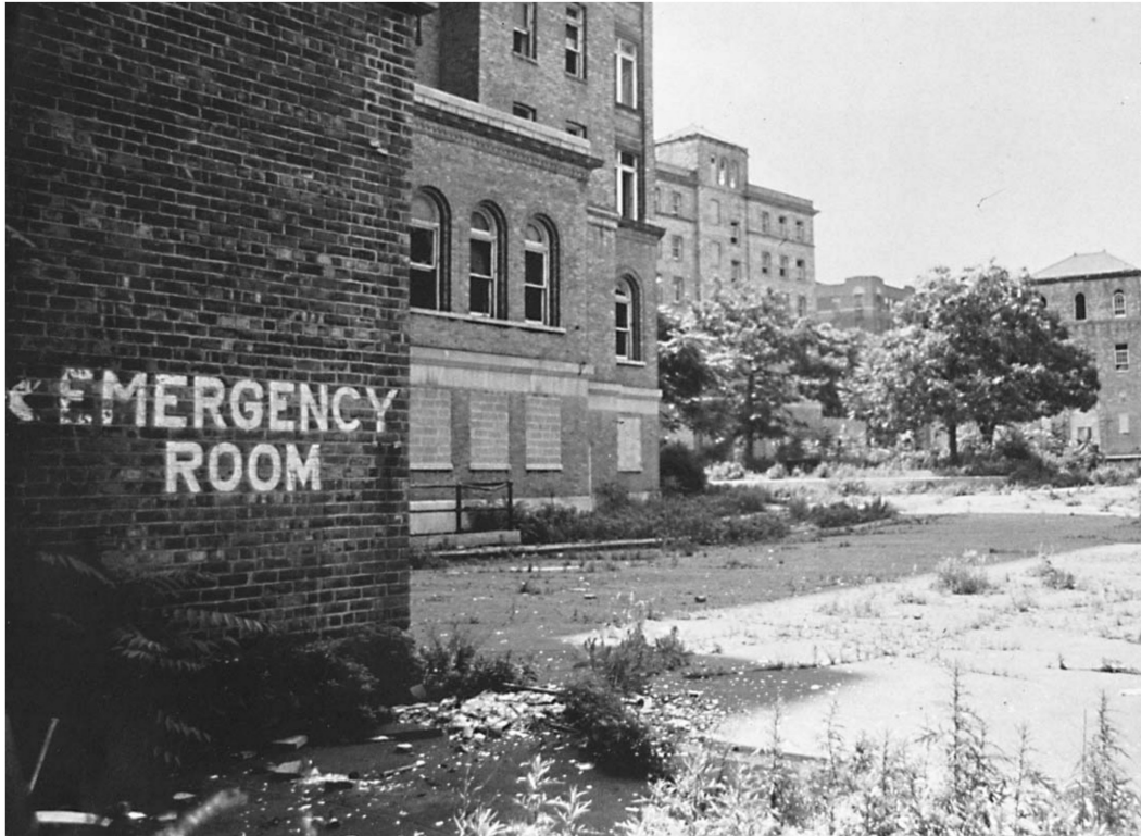
The collapse of urban infrastructure and health care are vital issues which were ignored by both leading Presidential candidates. Here, what used to be a hospital in New York's South Bronx.
