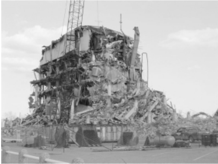
Production jobs gone, engineering jobs going. . . The Ford Engineering Center in Dearborn, Michigan was being demolished in March. Detroit's ambitious and well-educated school graduates, Representative Lemmons says, leave the city. Historical reverse-migration to the South is under way.
