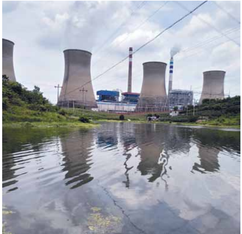
The Qianxi Power Station, a coal-fired power plant near Gantang, Guizhou Province, China.
