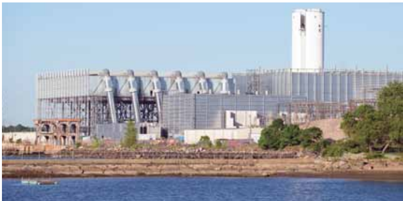
The Salem Harbor Natural Gas Power Station in Salem, Massachusetts.
