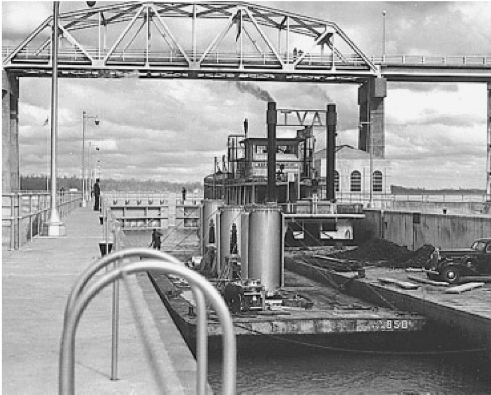
The Tennessee Valley Authority (TVA), the greatest project of the Roosevelt era, transformed that whole section of the southern United States. Here, the Wheeler Dam Navigation Lock in 1942.
